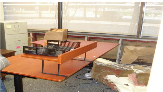
*As Ike battered the building, water leaked around the windows of Literacy Advance's headquarters on Wilcrest in Houston. Damage to the walls was significant and mold invaded carpet, furniture, and supplies.*
